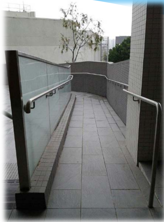
Ramps at hostel
