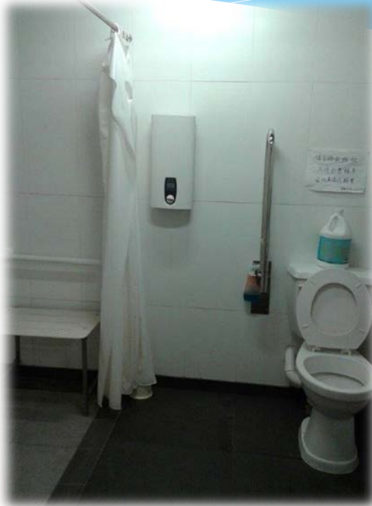
Shower room & toilets
